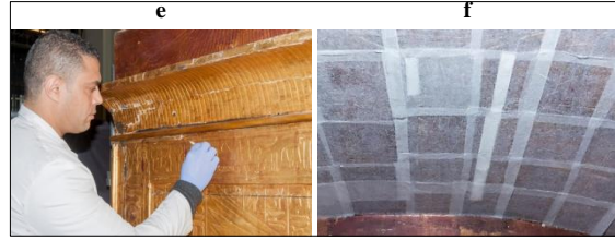
Figure (8) a, missing parts of the gilding layer in the east side due to the friction of opening and closing the doors, b, separating and flaking layers of the ceiling, c, paraffin wax layer agglomeration in the cracks, d, e, cleaning the ceiling and sides of the shrine, f, facing the interior ceiling.
