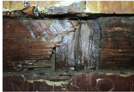
Figure (3) the inner frieze that was removed, showing part of a wooden tongue that joined the sides with the ceiling. Photo by authors
